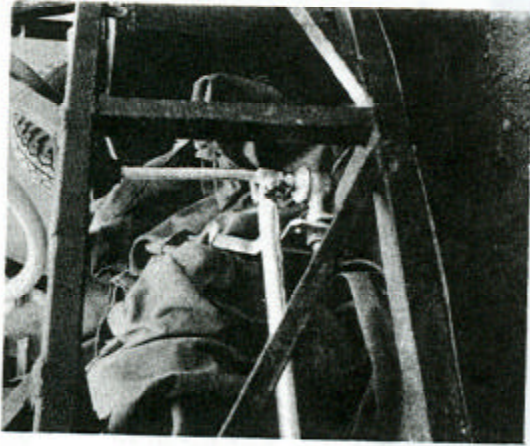
GEAR-SHIFT AND LOCK-OUT DEVICE. ADJUST FOR PROPER OPERATION.
